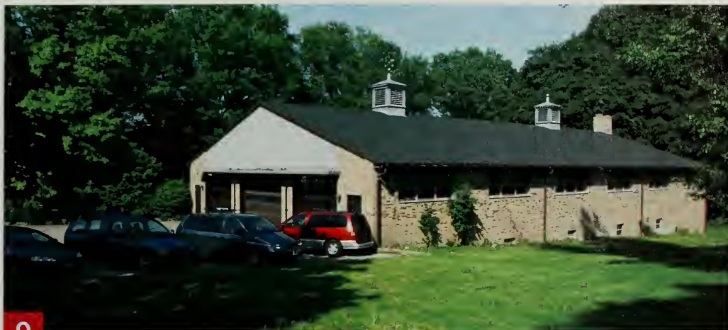
9 A two-level parking and storage facility beside the road to St. Clement's
